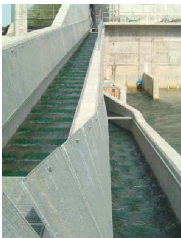
(2) Fish pass ramp
